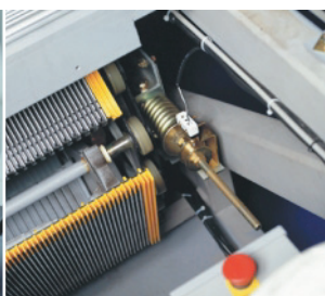
⑧ Step Chain Safety Device
